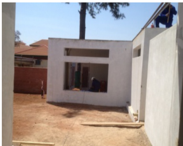
Tshwane District Hospital–TB ward: Plastering and basecoat
