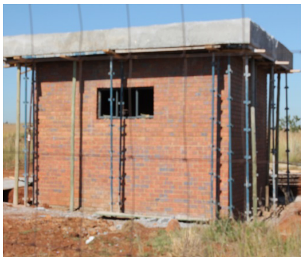
Suikerbosrand Northern Waterline – Installation of the Booster pump
