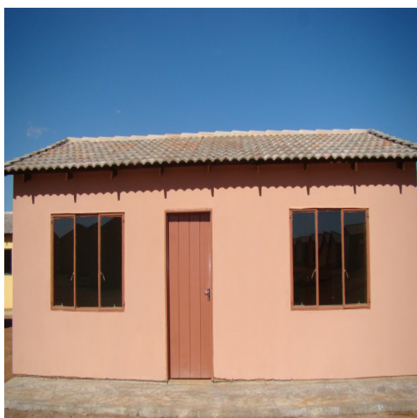
Albert Luthuli Housing Units
