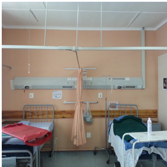
Edenvale Hospital additional oxygen and Vacuum points installation
